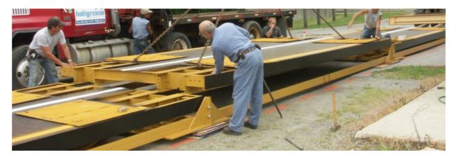
7. Install splice bolts on all 4 corners of the center section. Using the 56 ¾" x 2 ¼" bolts supplied. (14 per corner)
